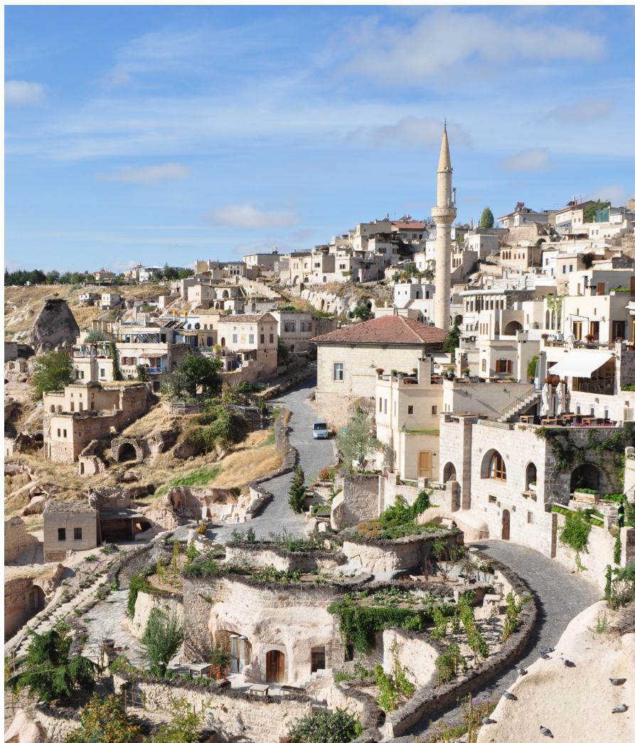
ABOVE: In order to preserve the landscape of Cappadocia, the region has strict rules for the restoration of buildings. The architecture of the building cannot be altered (walls may not be removed), and any new construction must use similar-colour stone of the existing building or tufa (limestone). Photo: Tracey Ho Lung BELOW: A surprisingly bright, cave-style room at the Ariana Sustainable Luxury Lodge in Cappadocia. Photo: courtesy of Ariana Sustainable Luxury Lodge
